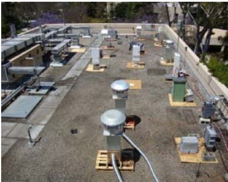
Roof top of CalTech (Pasadena)
